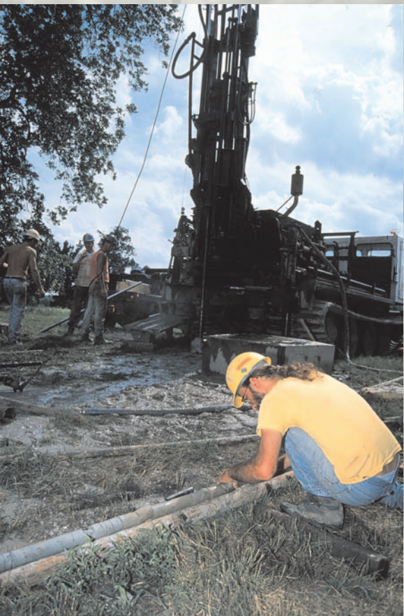
Geologist describing core from deep test boring
