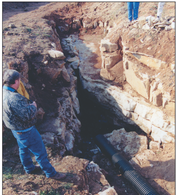
Figure 3 The excavation of a sinkhole reveals a long crevice in the exposed St. Louis Limestone bedrock that leads to a somewhat wider crevice. The wider crevice led down, about 15 feet, into a small cave about 0.3 m (1 foot) high and 0.6 m (2 feet) wide through which runoff from rainwater and snowmelt can flow. (Photographs by Samuel V. Panno.)
