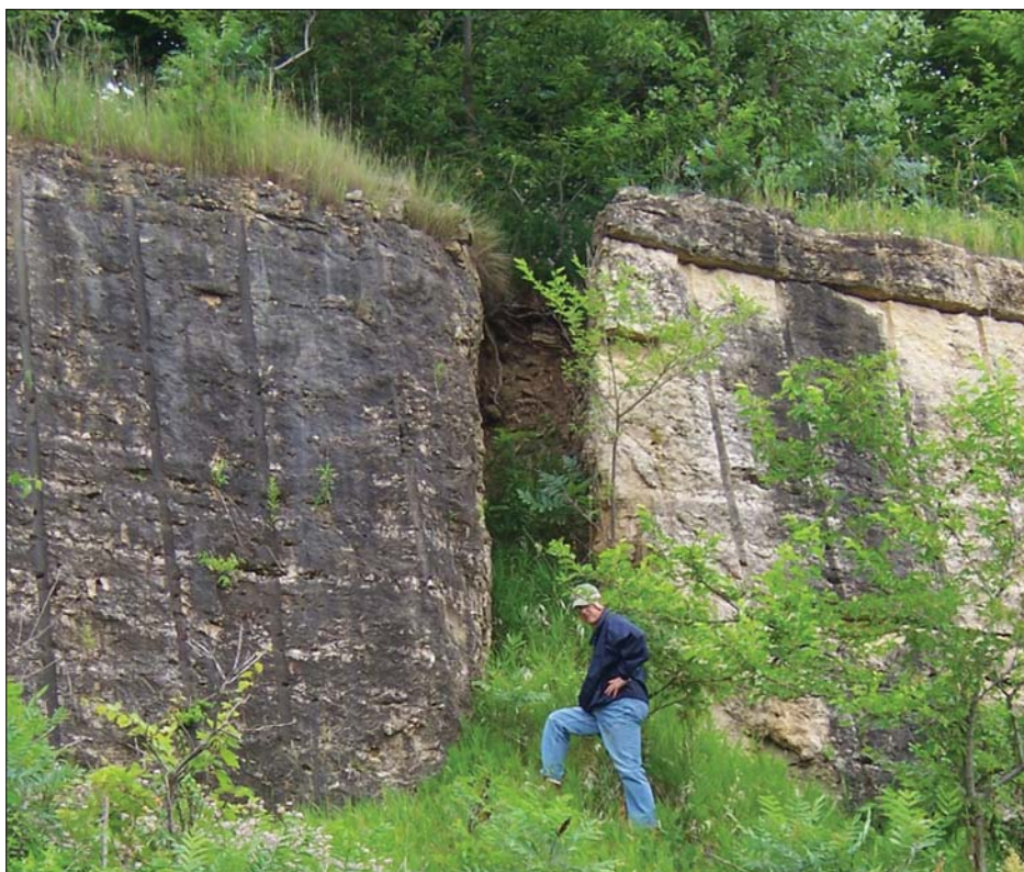
Figure 13 Road cut exposure of Silurian-age dolomite near Elizabeth, Illinois, in Jo Daviess County. Solution-enlarged crevices in the Silurian dolomite can be up to approximately 3 ft (1 m) in width (photograph by S. Panno).
